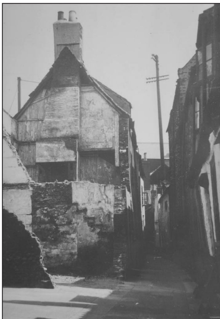
Row thirty, photo by P.E.Rumbelow
